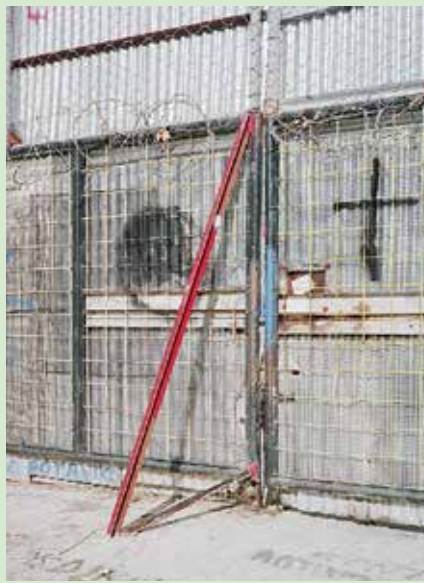
The entrance to the construction site of the new mosque in Votanikos. It's been more than a decade since a presidential decree gave the go-ahead for an official mosque in Athens © Antonis Theodoridis
